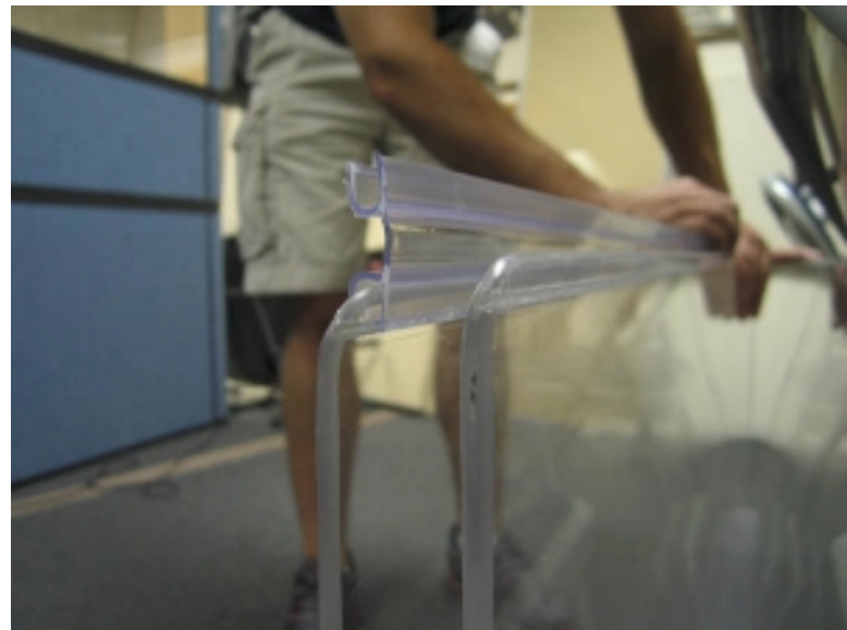
4. Continue seating hinge into groove
